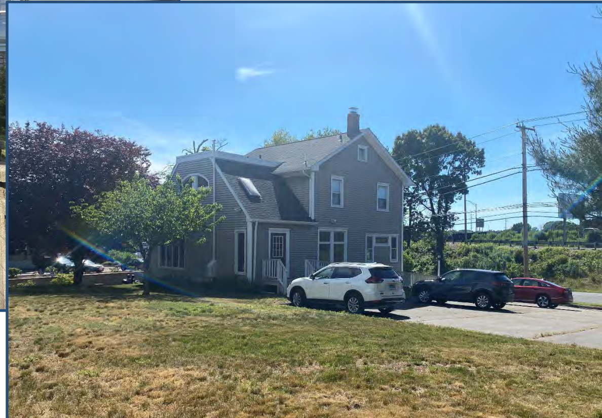
Rear Building and Parking
