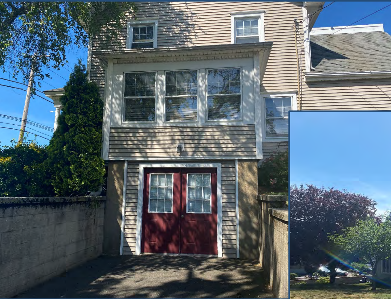
Lower Level Office Entrance
